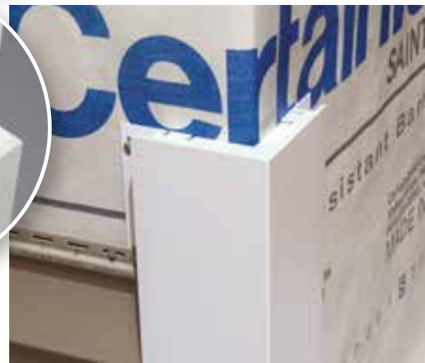
One-piece, smooth 6 in. corner with J-pocket, using flange installation.
